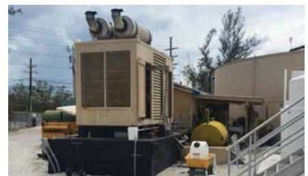
Kohler Genset Removed
